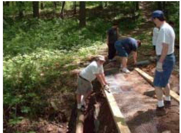
Warthog patrol working on bridge repair
