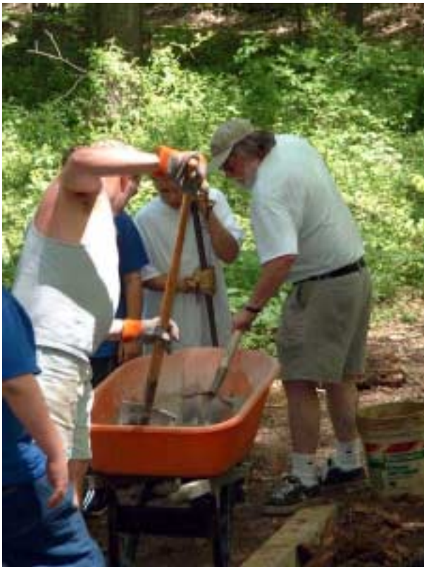
Mixing concrete
